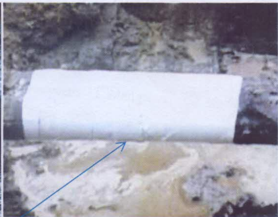
3mm Hacksaw cut on the Facility (Before & after repair)
