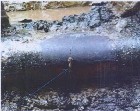
3mm Hacksaw cut on the Facility (Before & after repair)
